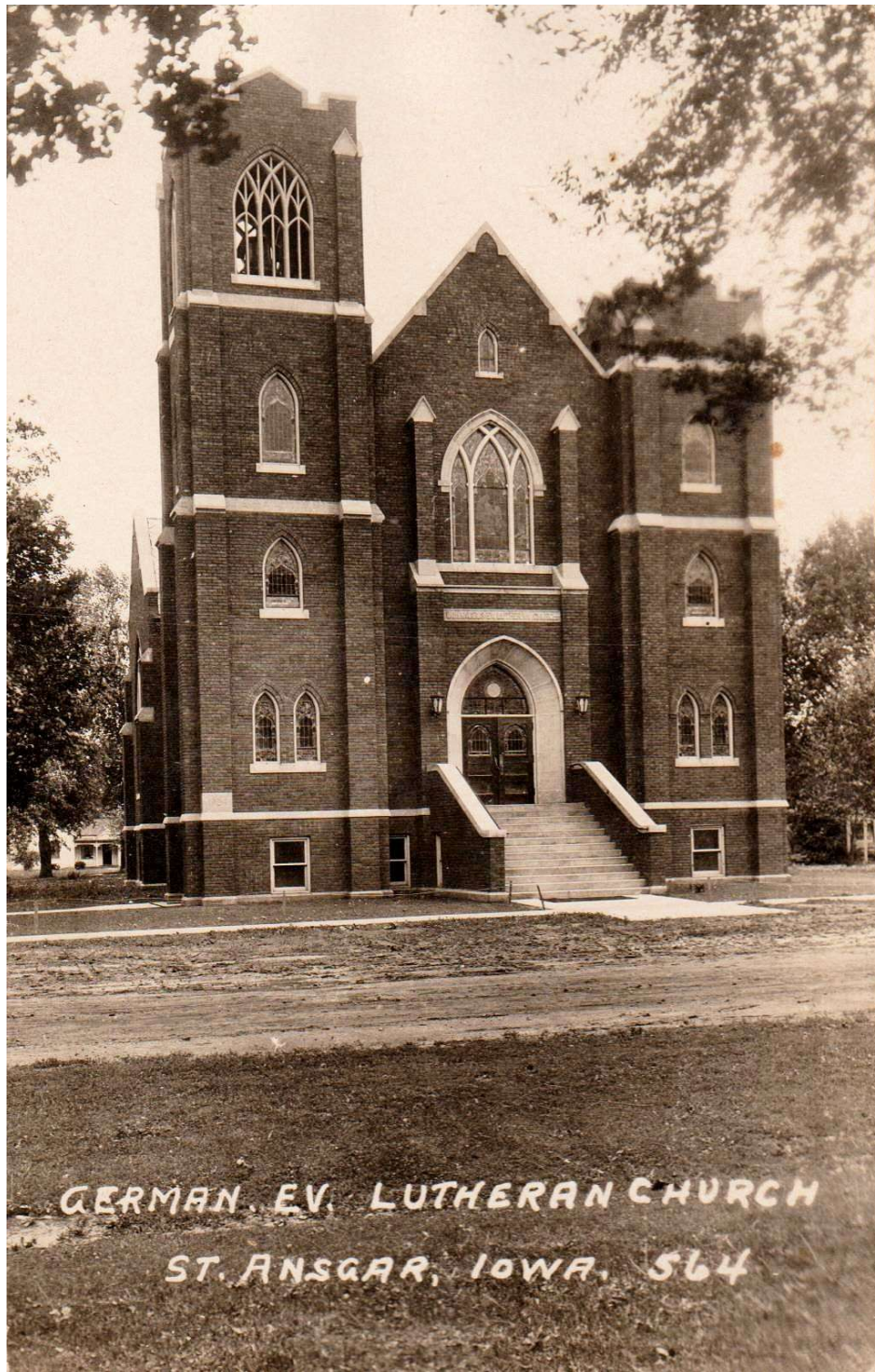
Brick by Brick Building of the New Church 1924
