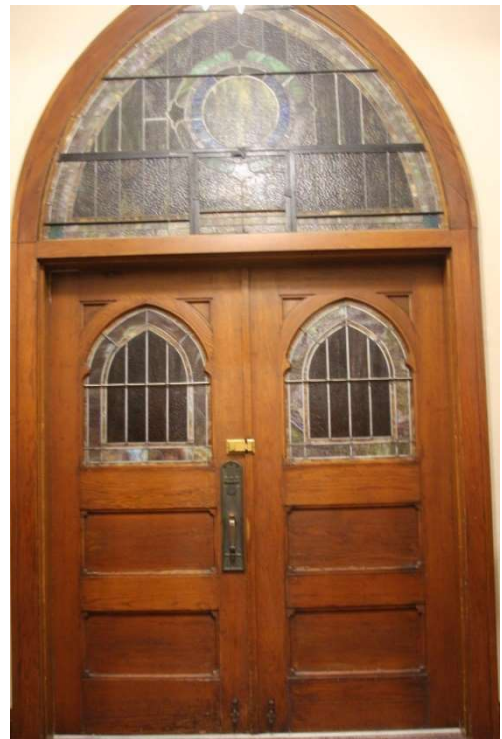
Main doors to the north, located in narthex
